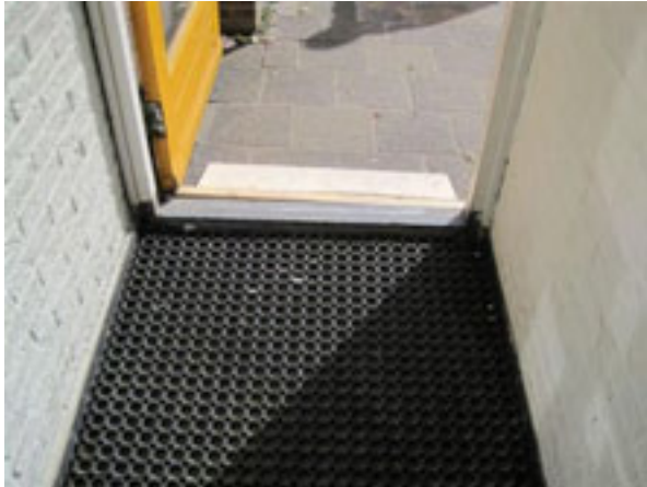
Gladde plank, smaller dan drempel. Noppenmat te stroef.
